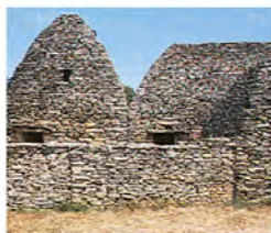
Bories (see p173) are drystone huts built using techniques dating back to 2,000 BC.
