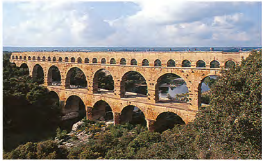
The Pont du Gard, the tallest of all Roman aqueducts at 48 m (158 ft)
