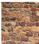
Roughly cut stone bricks are used to make the walls.
